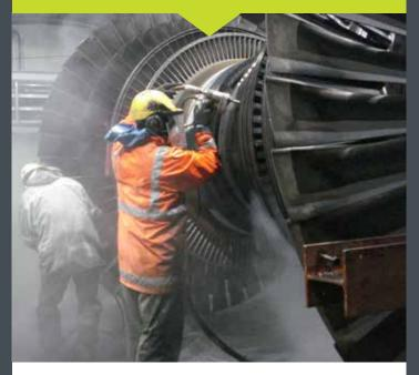
For thermal and geothermal power generation facilities, our unique low-flow rate, but ultra-high pressure pumps allow operators to tackle tight spaces and complex shapes such as cleaning ash from inside boilers or silica scale from turbine blades.
